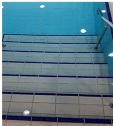
Figure 2. Pool Entry Steps
